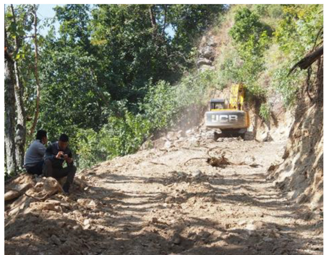
Fig. 7. Road construction to reach an integrated settlement in Tiru.
